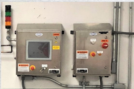
NEMA 4X Control Panel for wash down environment with water-shed design.
